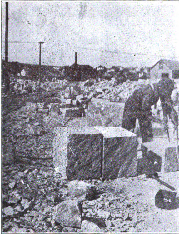
The Big Block Cut in Two with Wedges. This Requires Much Skill. Drilling with Compressed Air Drilling Machine.—From Vinalhaven, Maine.
